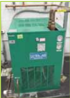
ULTRA AIR UA125 3/4 HP REFRIGERATED COMPRESSED AIR DRYER
