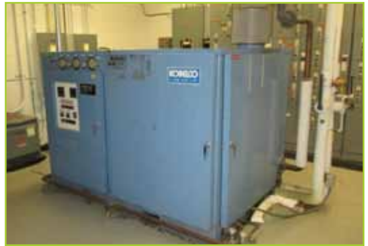
KOBELCO KNW1-A 100 HP ROTARY SCREW AIR COMPRESSOR
