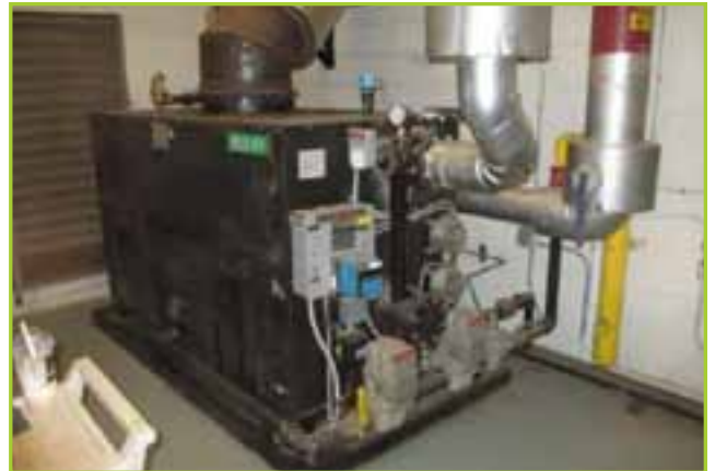
PARKER T2600 NATURAL GAS HOT WATER BOILER, MAX WORKING PRESSURE 150 PSI, HEATING SURFACE 337 SQFT, MAX STEAMING CAP WATER 2080 LB/HR OR MBH, BUILT 95 INSERT YR 2000
