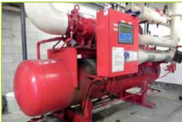
FES 200HP SCREW AMMONIA COMPRESSOR, MODEL: 180-HE, SN: 2052876, W/ CIRCULATION SYSTEM AND BAC EVAPORATIVE CONDENSER
