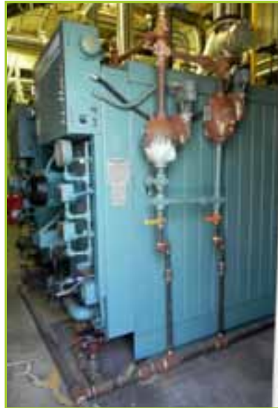
(2) CLEAVER BROOKS BOILERS, MODEL: M5P-6000LV
